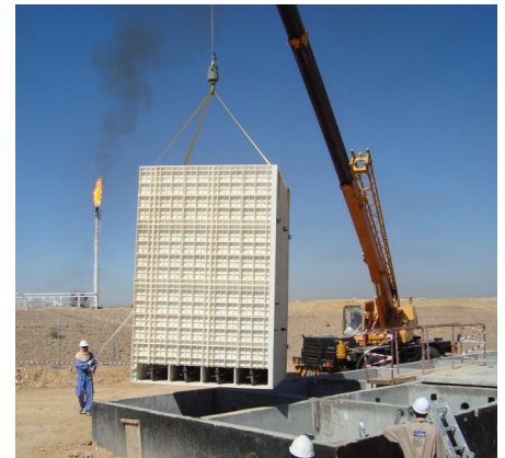
Installation of a BioReactor system in Yemen
