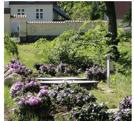
Mars 3000 installed at Boarding School
