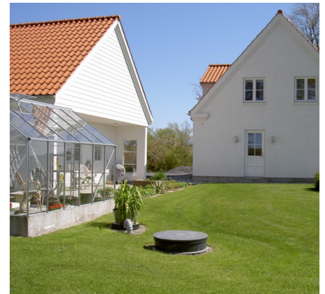
Pluto installed at a family house
